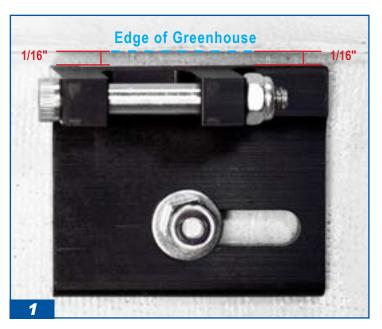
**STEP 2:** Begin with one side. With the latch unlocked, place the latch assembly into position over roof bolt. Press down on the latch assembly so that it locks and goes into place. Tighten the nylon locknuts just enough so that it stays in place.
